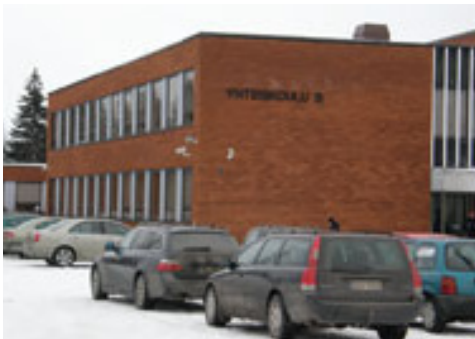
Avalarm Surveillance Installation Featuring Lumenera's Le175 Digital Camera
